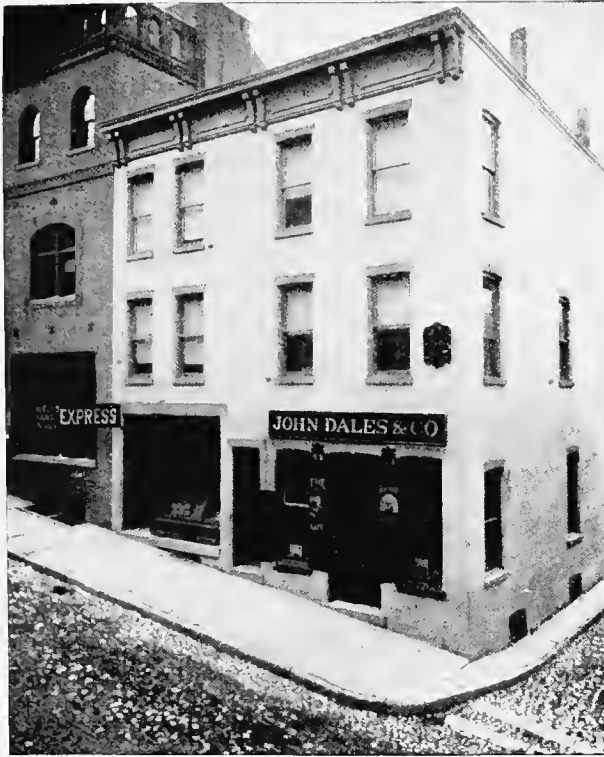
THE DALES BUILDING—44 and 46 Third Street.
